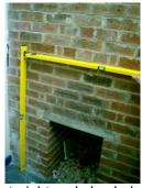
Check that the wall is straight and plumb, by using a spirit level as shown. If the wall is not plumb or is bowed, then the fireplace may not fit correctly
