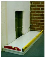
Place the hearth on top of the bedding mixture and locate to the pencil marks. Tap the hearth down gently until it is level and raised off the floor by approximately 5 to 10mm. Use spirit levels to check
